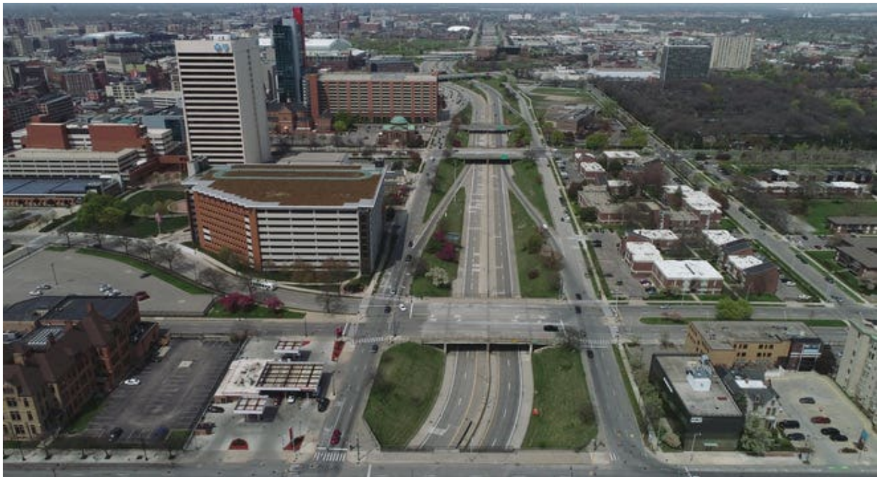
A view of Interstate 375 through downtown Detroit on April 23, 2021. The Michigan Department of Transportation is working on plans to replace I-375 with a boulevard because it is at the end of its useful life. Kelly Jordan and Mandi Wright, Detroit Free Press
